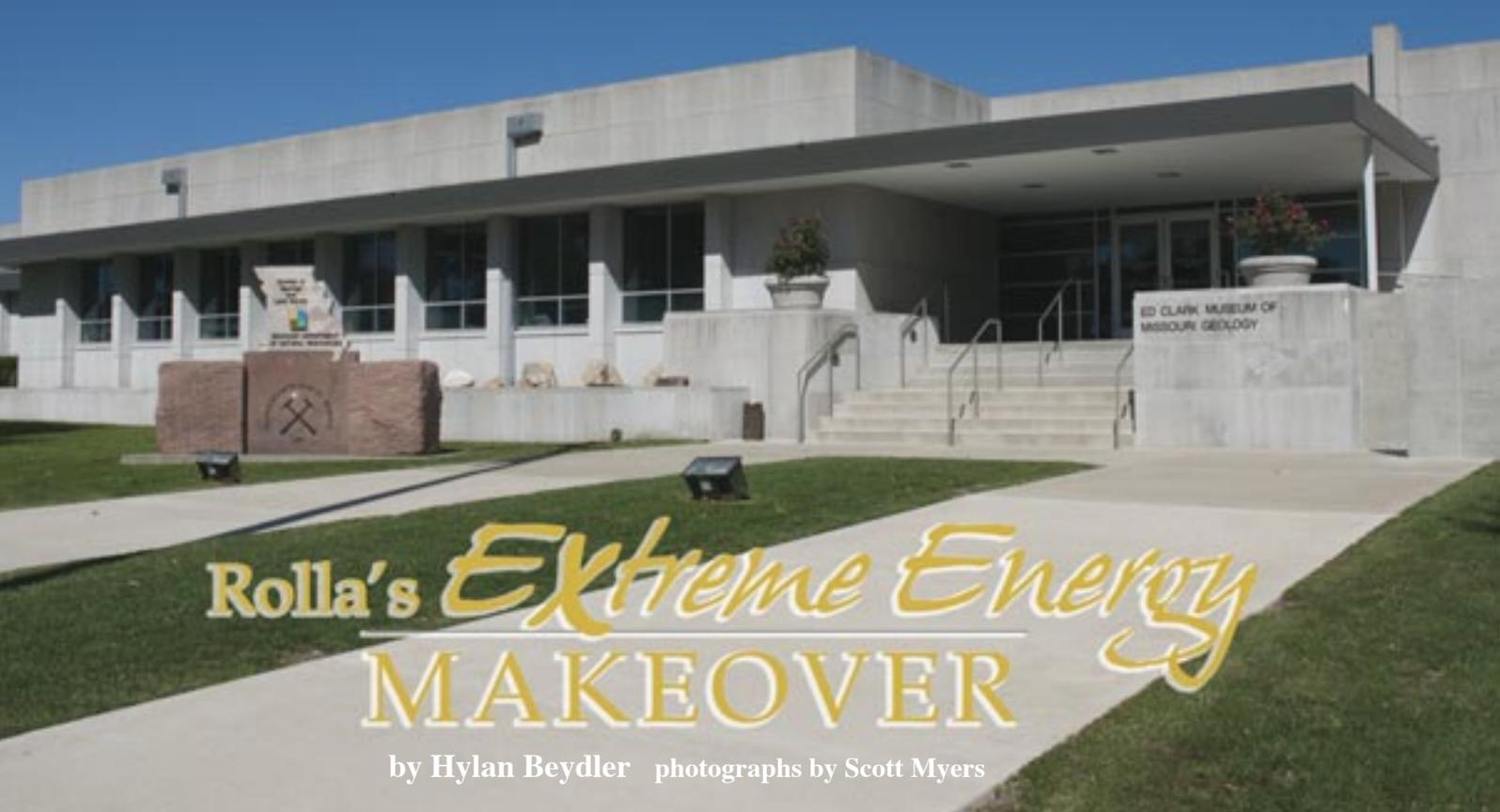
(Above) The Buehler Building, along with the DGLS Annex, not pictured, are two of the most energy-efficient buildings operated by Missouri state government. (Below) Double-pane, solar Low-E windows help increase energy efficiency. The building's overhang, part of its 1963 design, shades the windows in the summer and allows natural light into the building during winter months.
