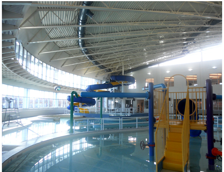
ARC pool area
