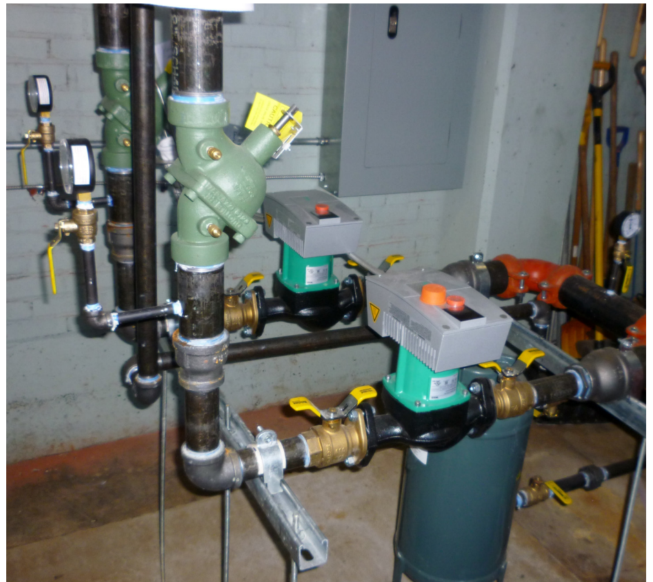
Above: One-pipe system requires less pumping power, fewer parts, is easier to maintain Left: Console heat pump units provide quiet comfort
