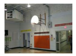
Fairview Elementary was retrofitted in the summer before the 2006-2007 school year. We replaced the heating system with our One-Pipe geothermal exchange system and added air conditioning and individual temperature controls to every space in the building. Energy consumption was slashed and comfort levels were dramatically improved. The installation cost was a low \$16.25 per square foot.
