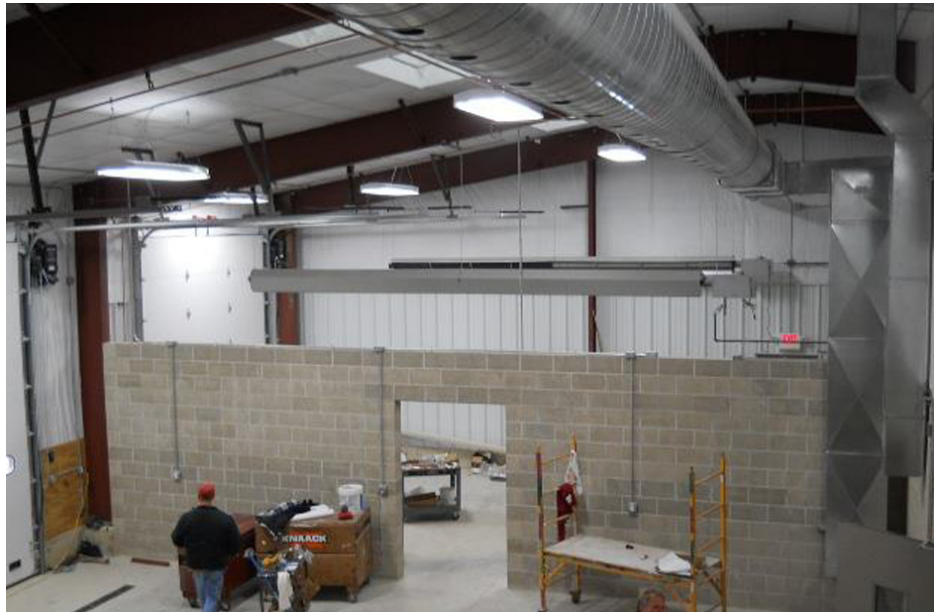
One of three maintenance bays
